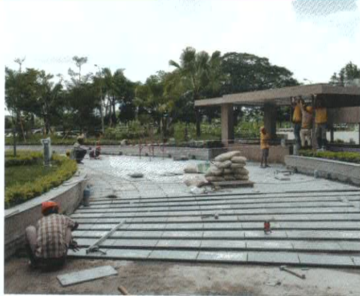
Many building materials are imported to Myanmar, driving up costs
