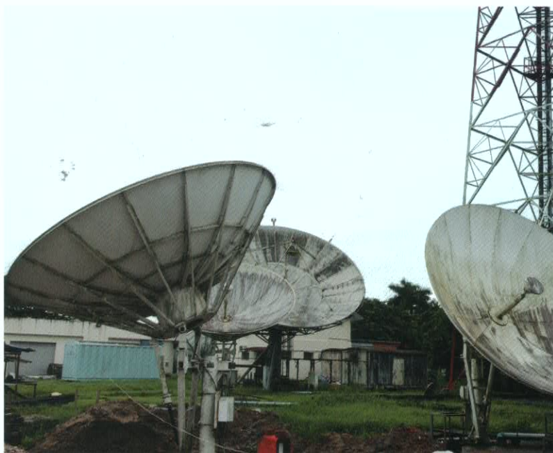
The expansion of communications infrastructure is critical to the sector's growth throughout the country
