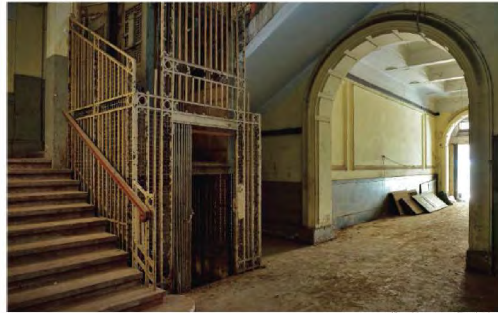
View of the entrance, lift and staircase
