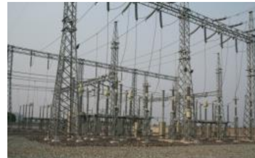
230 kV Kampot Substation (Cambodia)
