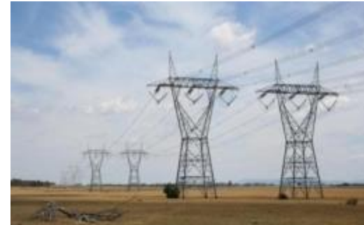
110kV / 220kV / 500kV Transmission Line projects (Vietnam)
