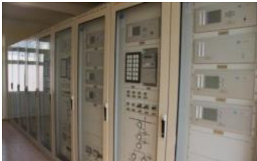
500kV CSCS Hiep Hoa (Vietnam)
