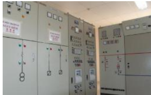
110 kV CSCS GS project (Cambodia)
