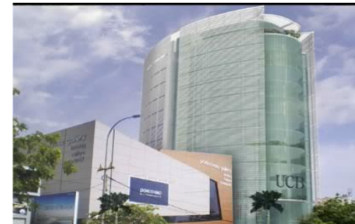
UCB Tower - Data Center (Cambodia)
