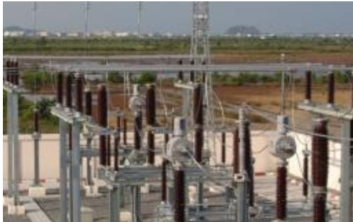
110 kV Substation Holcim Cement Plant (Vietnam)
