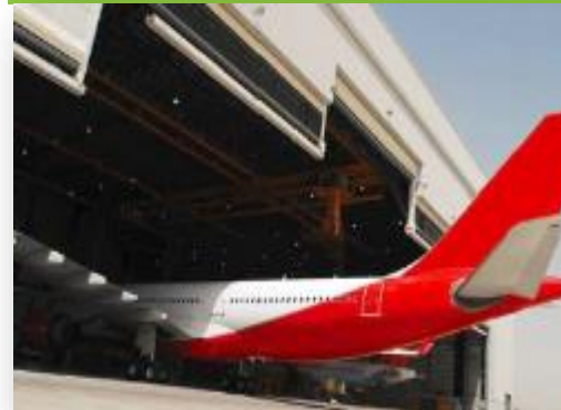
Naga World FBO Hangar (Cambodia)
