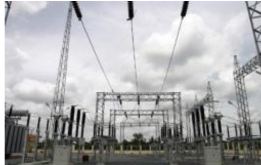
110kV / 220kV / 500 kV Transmission Substation projects (Vietnam)
